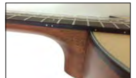
14th fret heel to body connection
